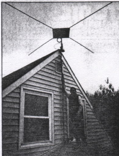
Photo G. The finished antenna.
